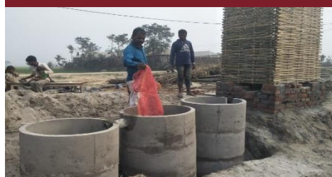
Low Cost and Sustainable constructed Toilets under FINISH Program with bamboo
