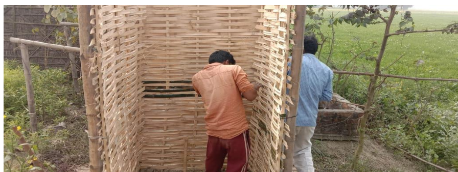
Low Cost and Sustainable constructed Toilets under FINISH Program with bamboo
