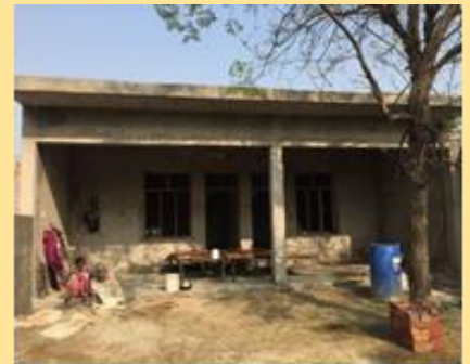
Fig. 3 Refurbished house of N Kaur
