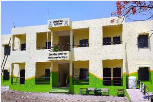
Fig. 6: Infrastructural Work in Ranjangaon School
